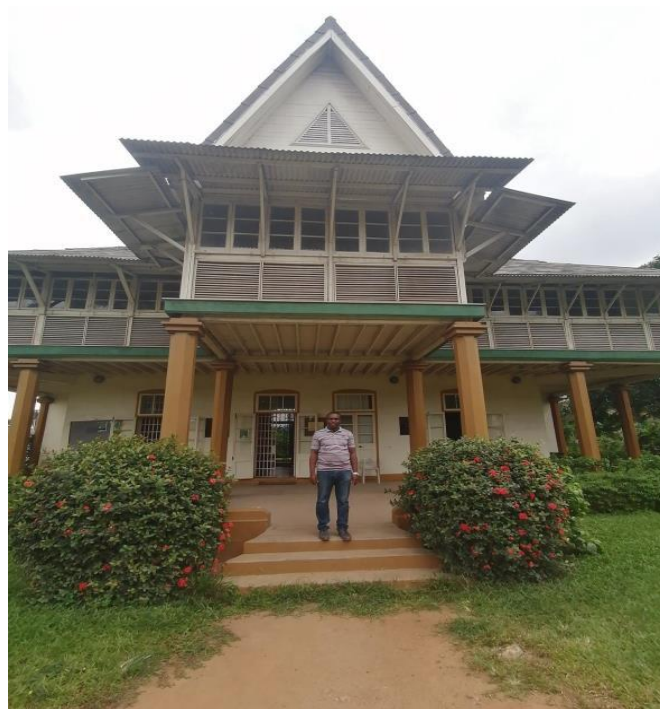
Figure 2. Front view of the Heritage Building with its distinctive architectural elements preserved in their natural state. Source: Author 2022.
